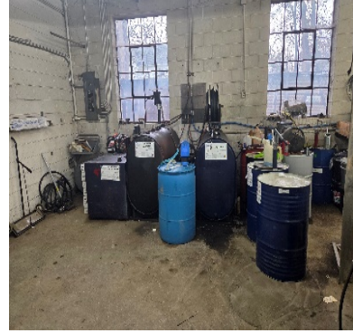
Bulk oil system — plumbed throughout shop Digital counter meters on every hose.
