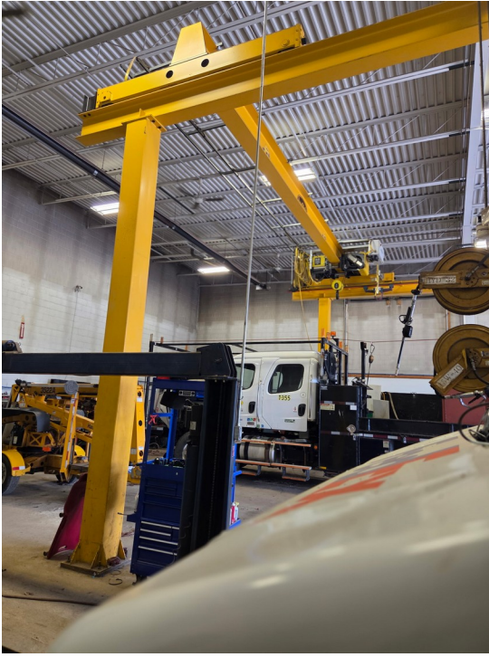
Rear Shop Workspace
